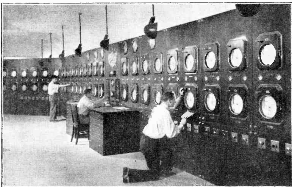
RADIO CITY, NEW YORK, is equipped with this special Air Controlling Plant, whereby the ventilation of each studio can be checked at any moment and changed to suit requirements. There are 64 dials. It is stated that four generators in the basement can produce "900 tons of refrigeration in 24 hours."
