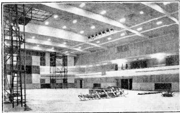
THE WORLD'S LARGEST STUDIO? Here is a portion of the huge "Auditorium Studio" in Radio City nearing completion. It measures 132 x 78ft. and is three storeys in height. The studio can accommodate 1,000 visitors and a 100-piece orchestra.
